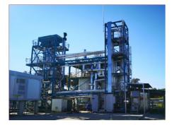
Power: **1.8 MWth** @ **14.0 MPa / 560 °C** Economizer/evaporator, air cooled condenser, pressure reducing station
