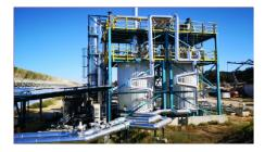
2-Tank TES 34 m3 (ca. 92 tons salt) Capacity: **5.4 MWh** @ **565 °C / ΔT = 275 K**
