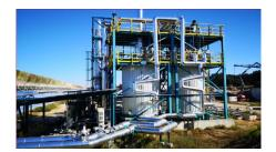
2-Tank TES 34 m3 (ca. 92 tons salt) Capacity: **5.4 MWh** @ **565** °C /  $\Delta$ T = **275** K
